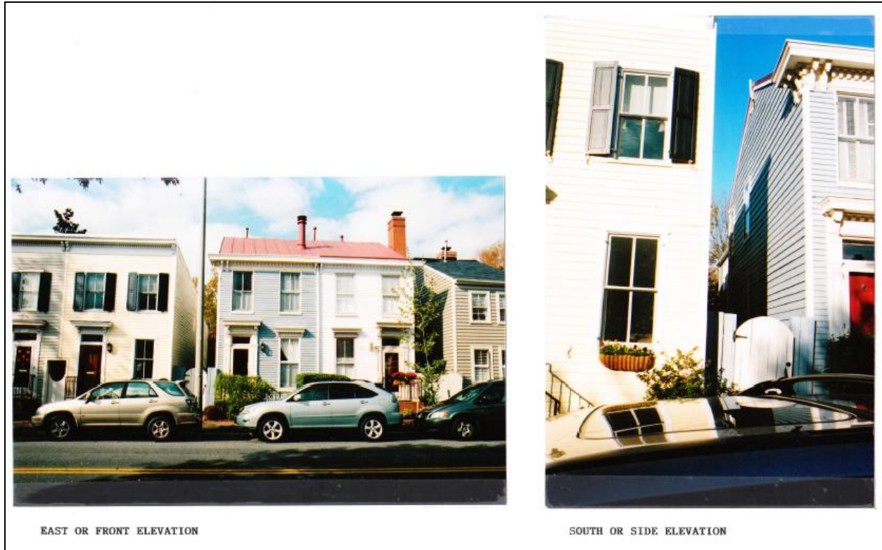
Figure 1. East (front) elevation and south (side) elevation.
