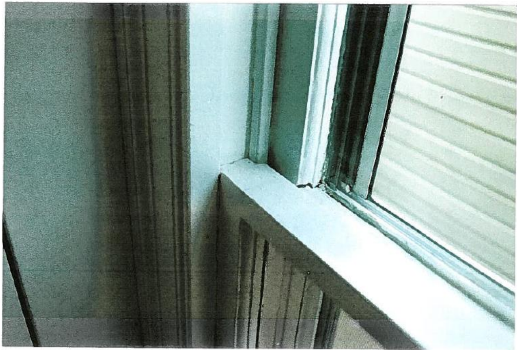
INTERIOR VIEW OF WINDOW SASH AT JAMB
