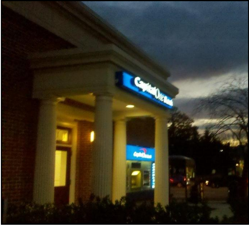
Figure 13: Photo of existing illuminated walk-up ATM.
