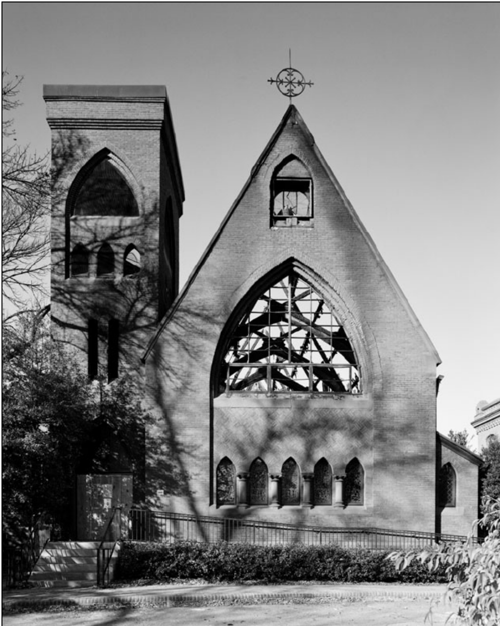
Figure 1. Existing conditions: east elevation.
