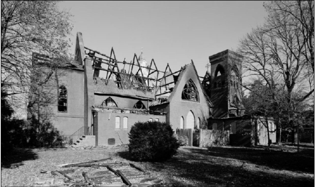
Figure 9. Existing conditions, south elevation.
