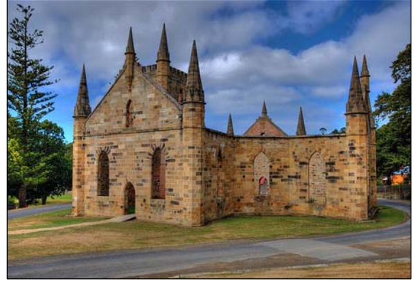
Figure 6. Port Arthur Church, Tasmania, Australia
