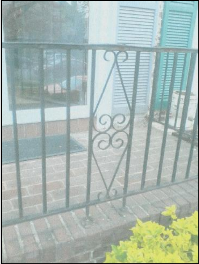
Figure 4. Detail view of Existing Wrought Iron Railing
