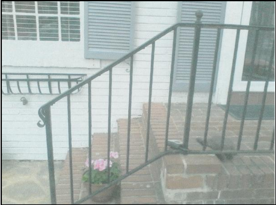
Figure 6. Existing Wrought Iron Railing
