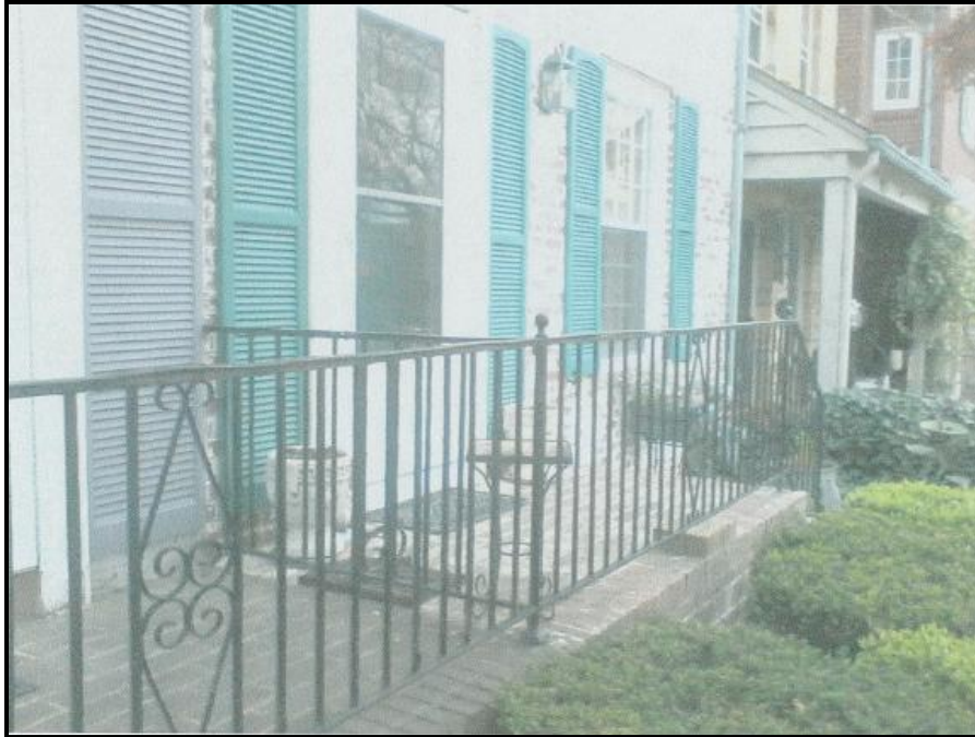
Figure 8. Existing Front Stoop
