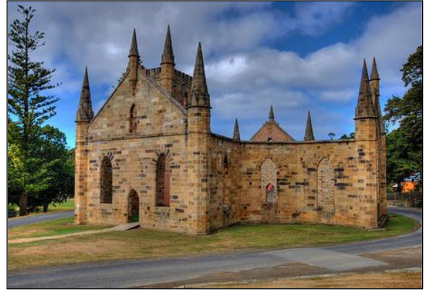
Figure 6. Port Arthur Church, Tasmania, Australia
