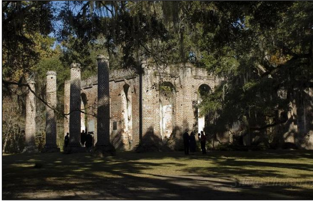
Figure 5. Old Sheldon Church, South Carolina
