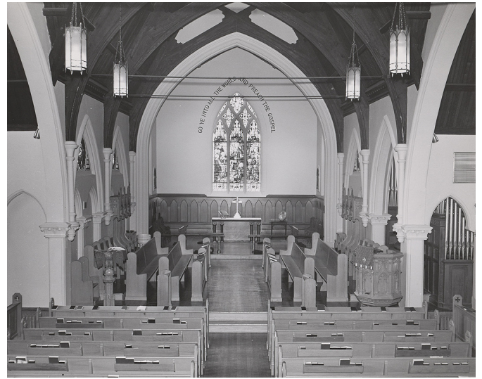
Figure 9: Interior post 1955 renovations
