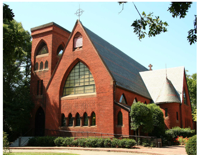
Figure 10: East Facade with accessible ramp, 2008
