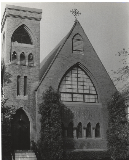
Figure 9: East Facade after loss of tower roof and alteration to upper lancet windows, c. 1990 before addition of accessible ramp
