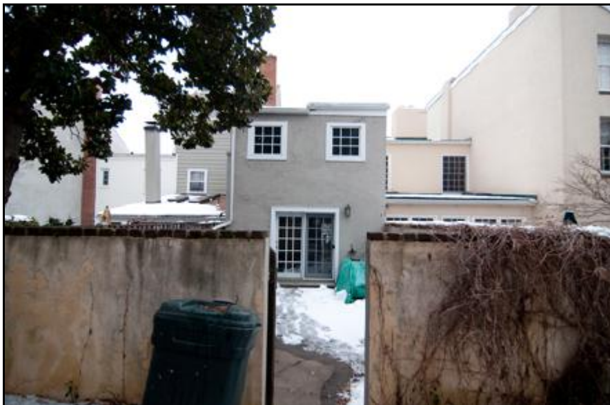
Figure 3: Existing Photo - Rear
