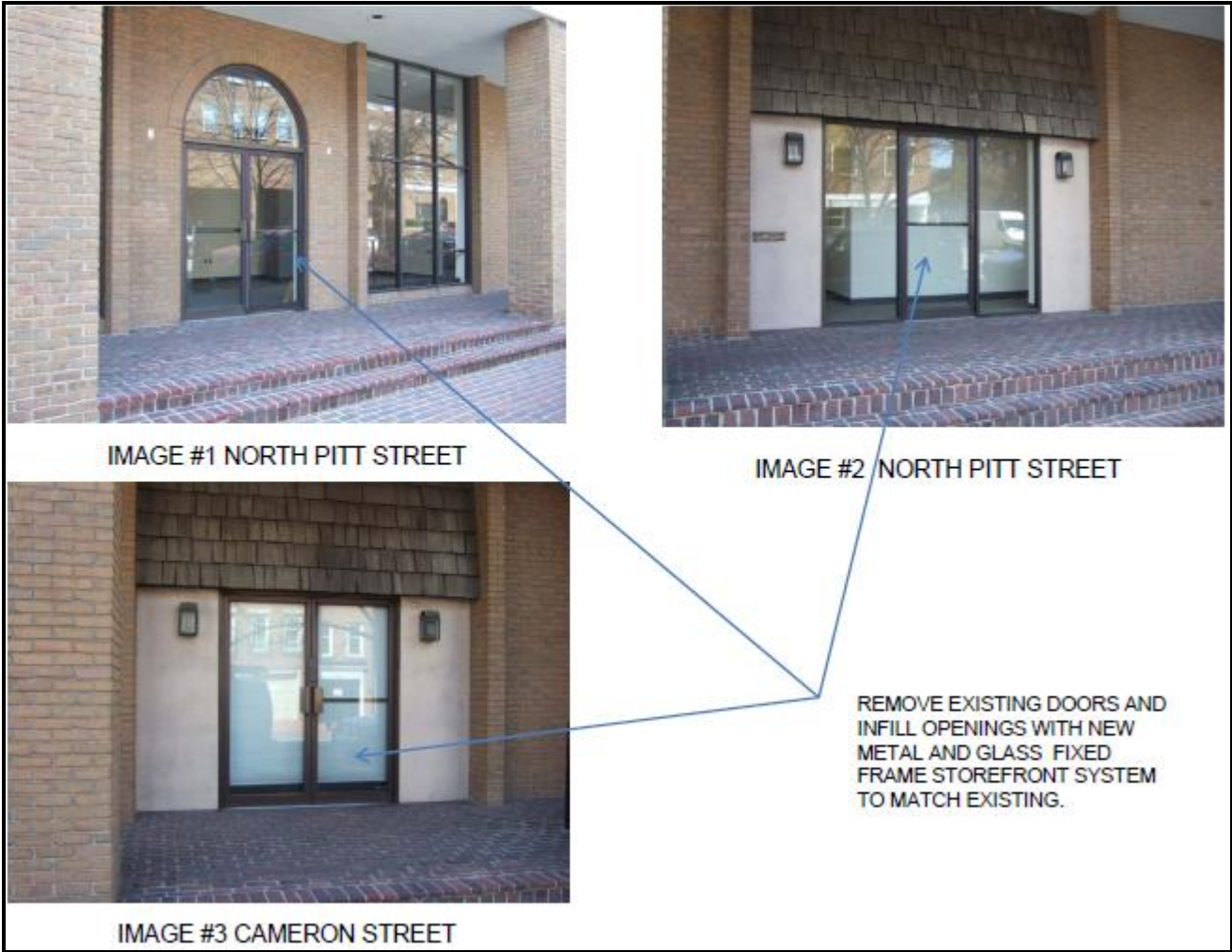
Figure 1. Photos of three existing entrance doors.
