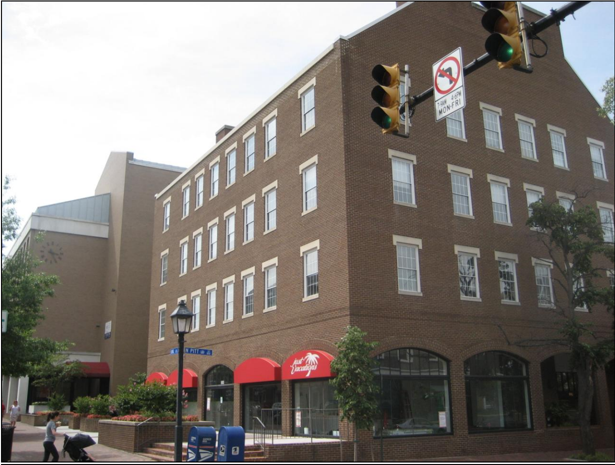
Figure 1. Looking northwest, south (front) elevation and east (side) elevation.
