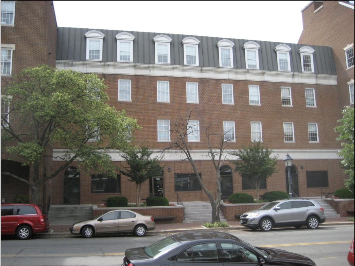
Figure 2. Rear portion of east (side) elevation.
