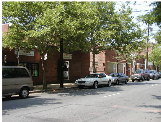
North End of Subject Block
