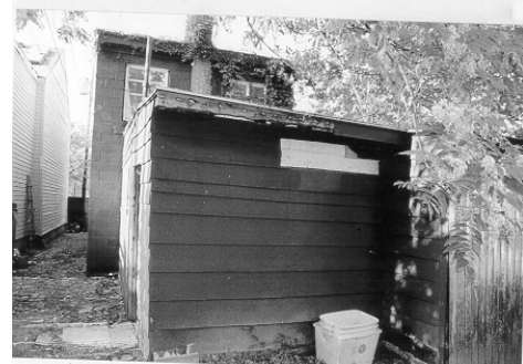
Figure 2 - East Side and Rear
