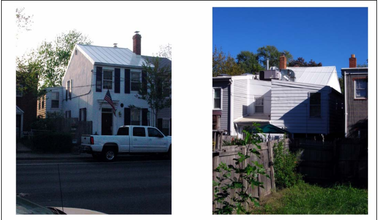
Figure 2. Existing conditions, 320 N. Patrick Street
