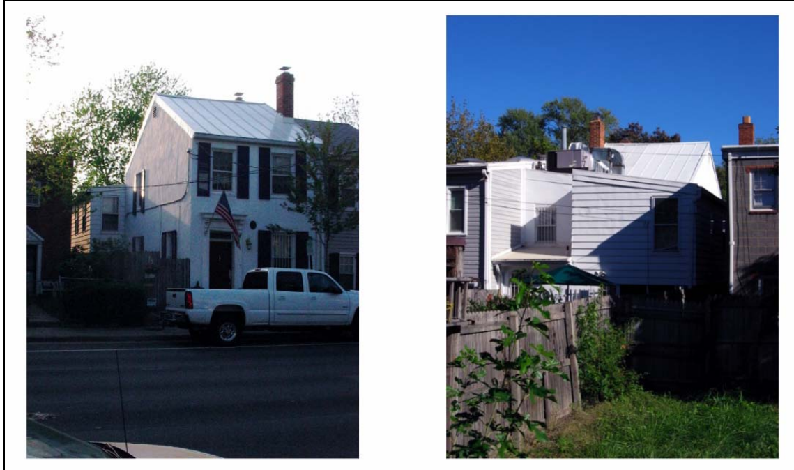
Figure 2. Existing conditions, 320 N. Patrick Street
