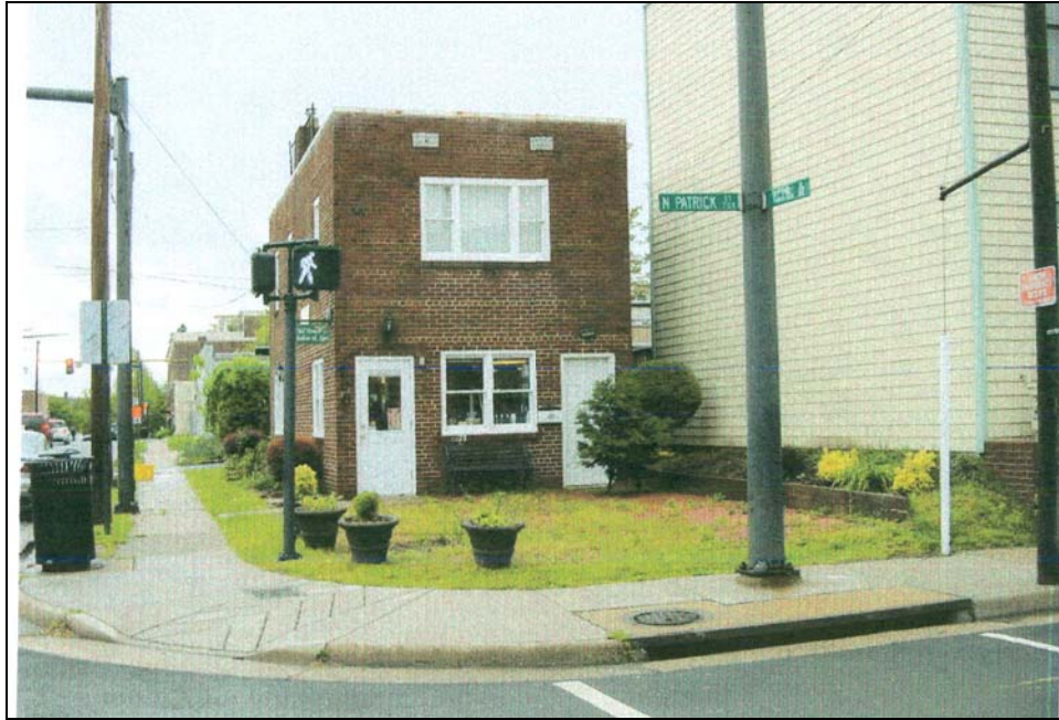
Figure 1. 700 N. Patrick Street, east elevation.
