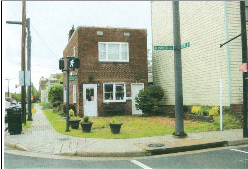
Figure 1. 700 N. Patrick Street, east elevation.
