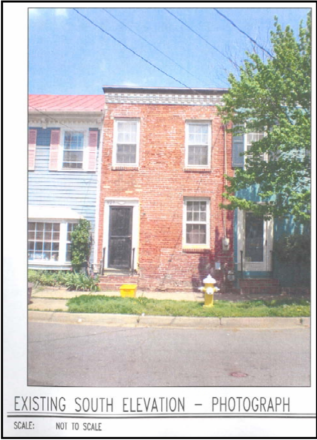
Figure 1 Photograph of Existing South Elevation
