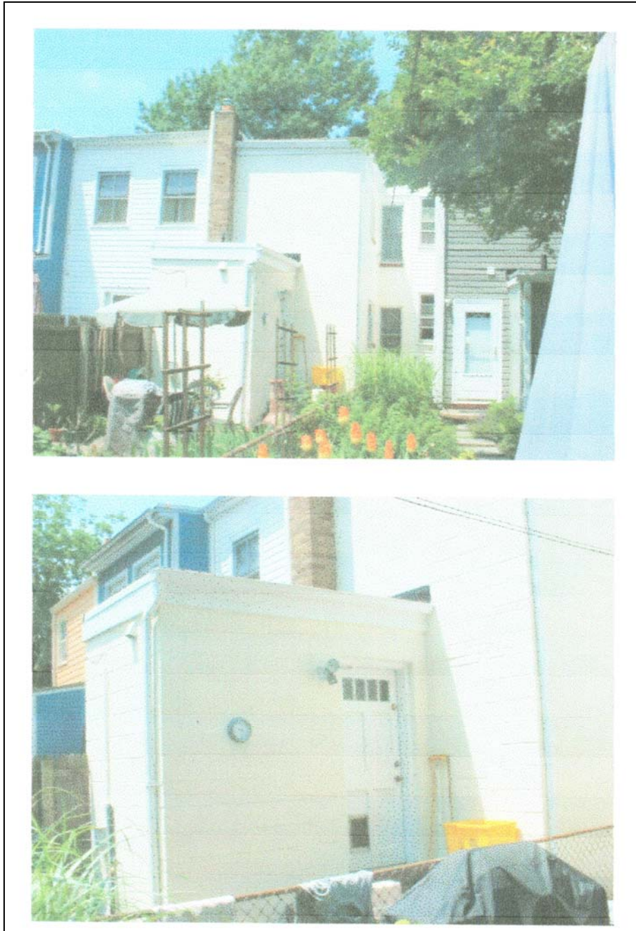
Figure 1: Rear of 309 North West Street, area proposed for encapsulation.
