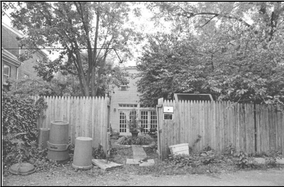
Figure 3: Existing rear elevation showing HVAC unit location
