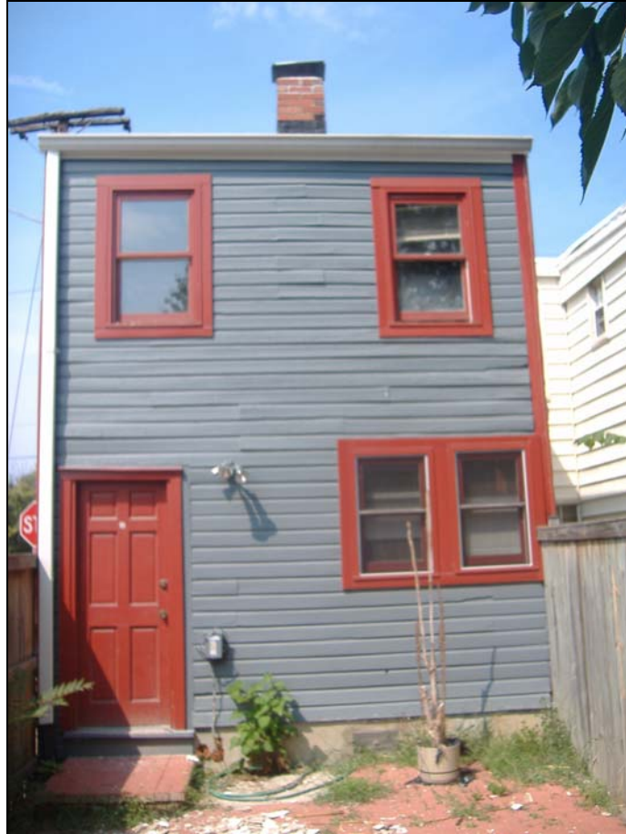
Figure 3. Existing rear (south) elevation.
