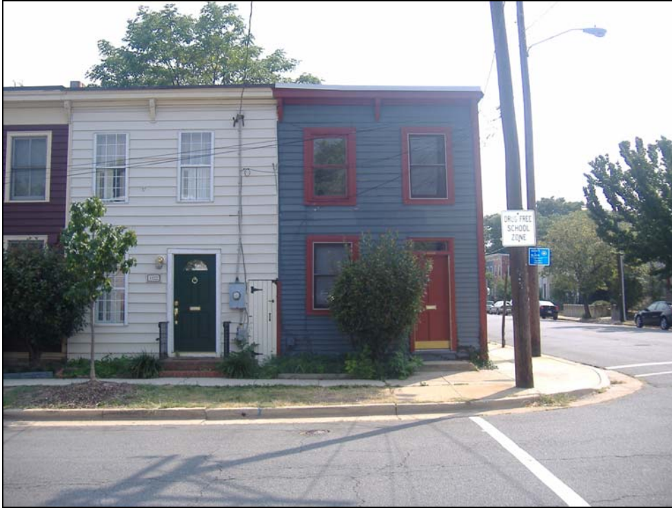
Figure 1. Existing front (north) elevation.
