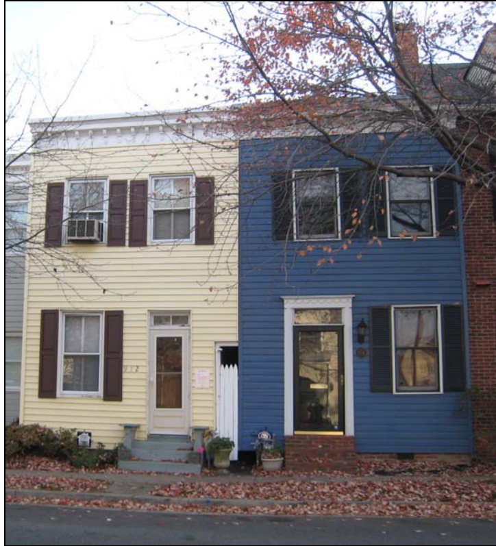
Figure 1. Front (north) elevation of 912 Pendleton Street (on left).
