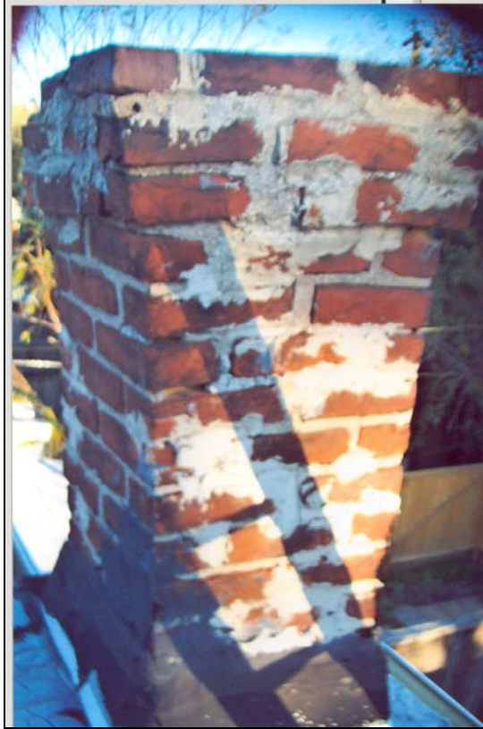
Figure 3. Detail of existing chimney.
