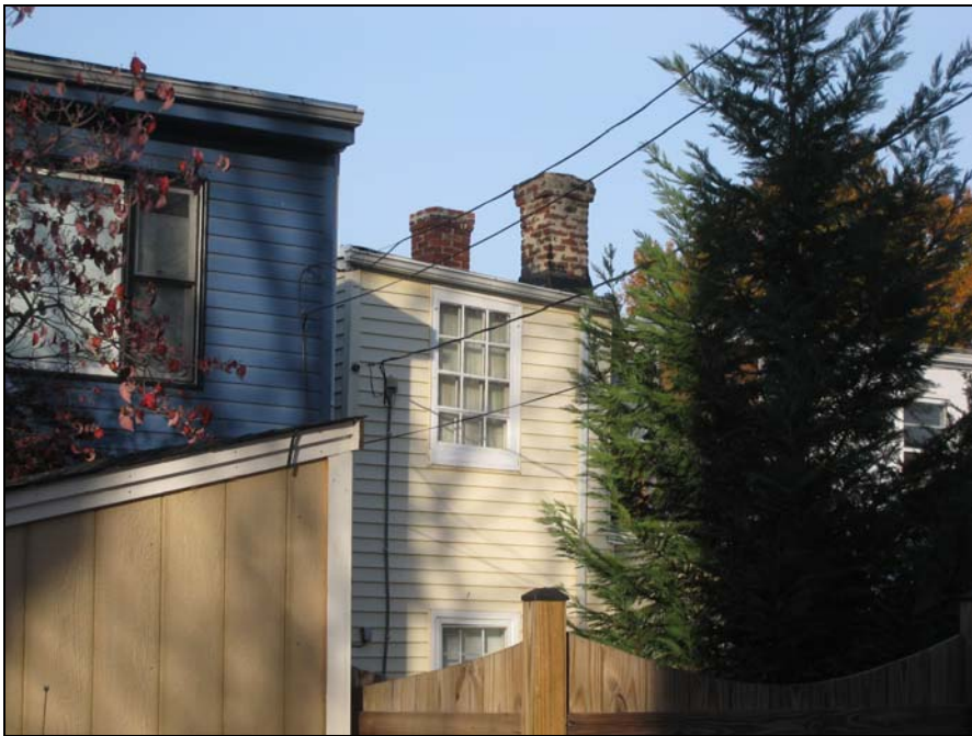
Figure 2. Rear (south) elevation with existing chimney.
