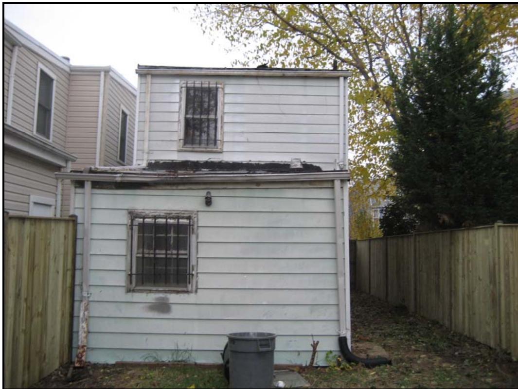
Figure 3: Photo of one story addition and upper second story wall to be demolished
