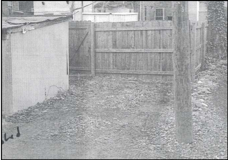
Figure 2: Photograph of yard with existing shed
