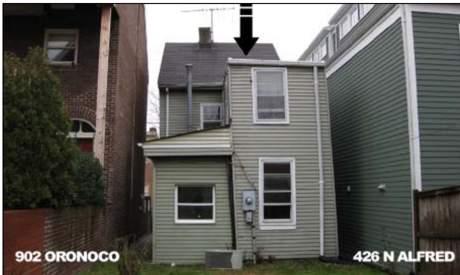
Figure 2. West elevation, 426 North Alfred Street.
