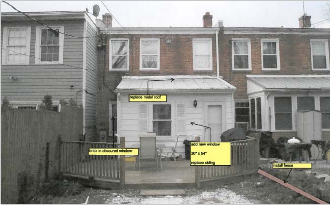
Figure 1. Existing conditions and proposed alterations on rear elevation: window to be bricked in and new opening to be created on one-story frame portion.
