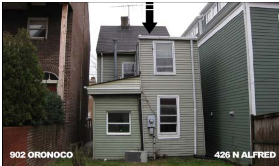
Figure 2. West elevation, 426 North Alfred Street.
