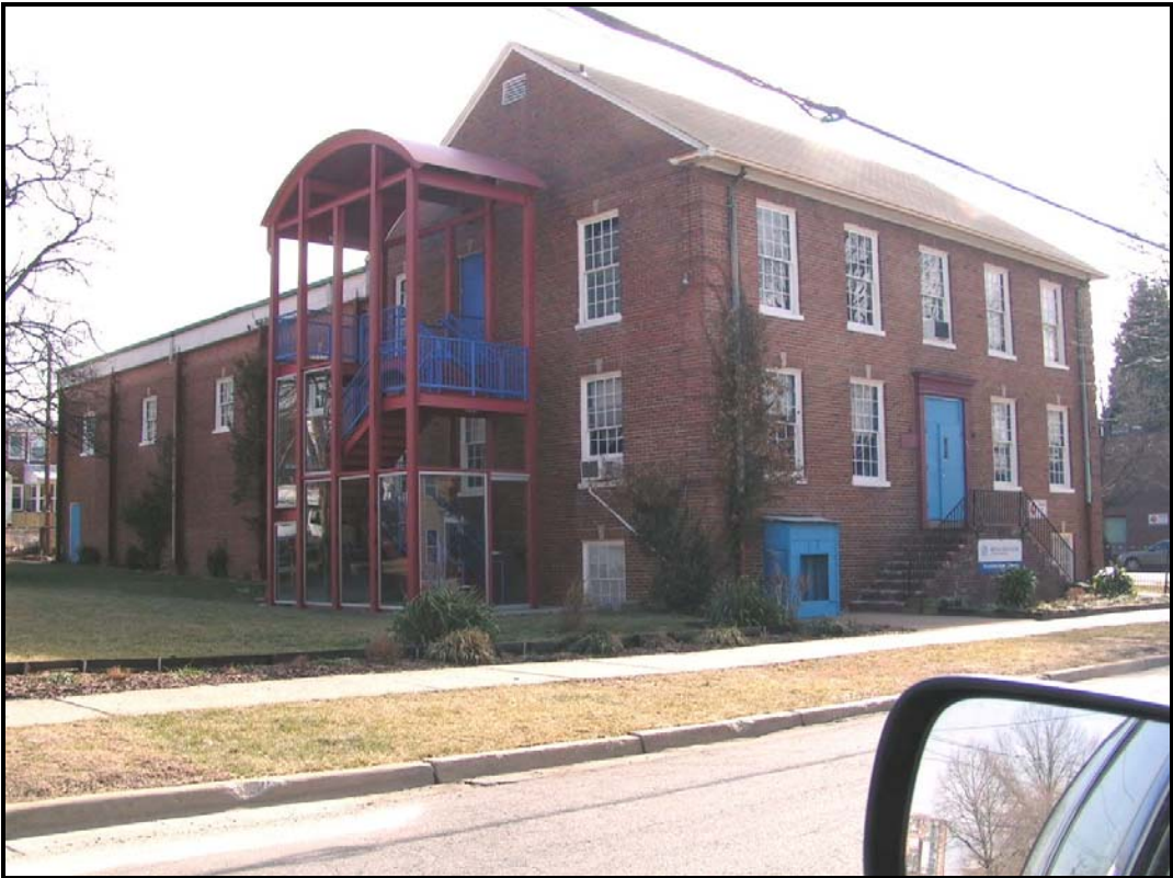
Figure 2. Photo of west and north elevations
