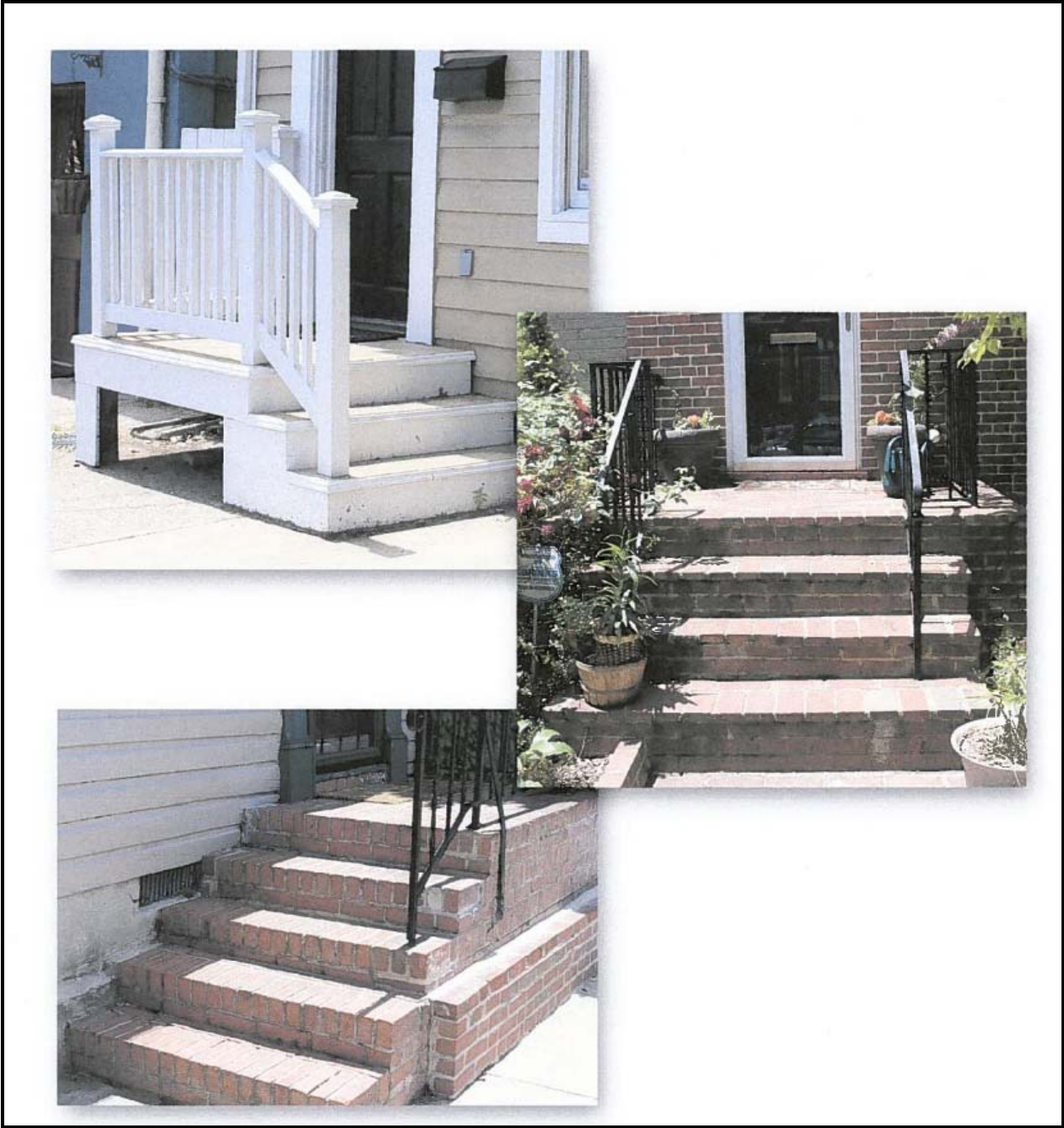
Figure 6. Photos of stoops and railings in the Parker-Gray neighborhood.
