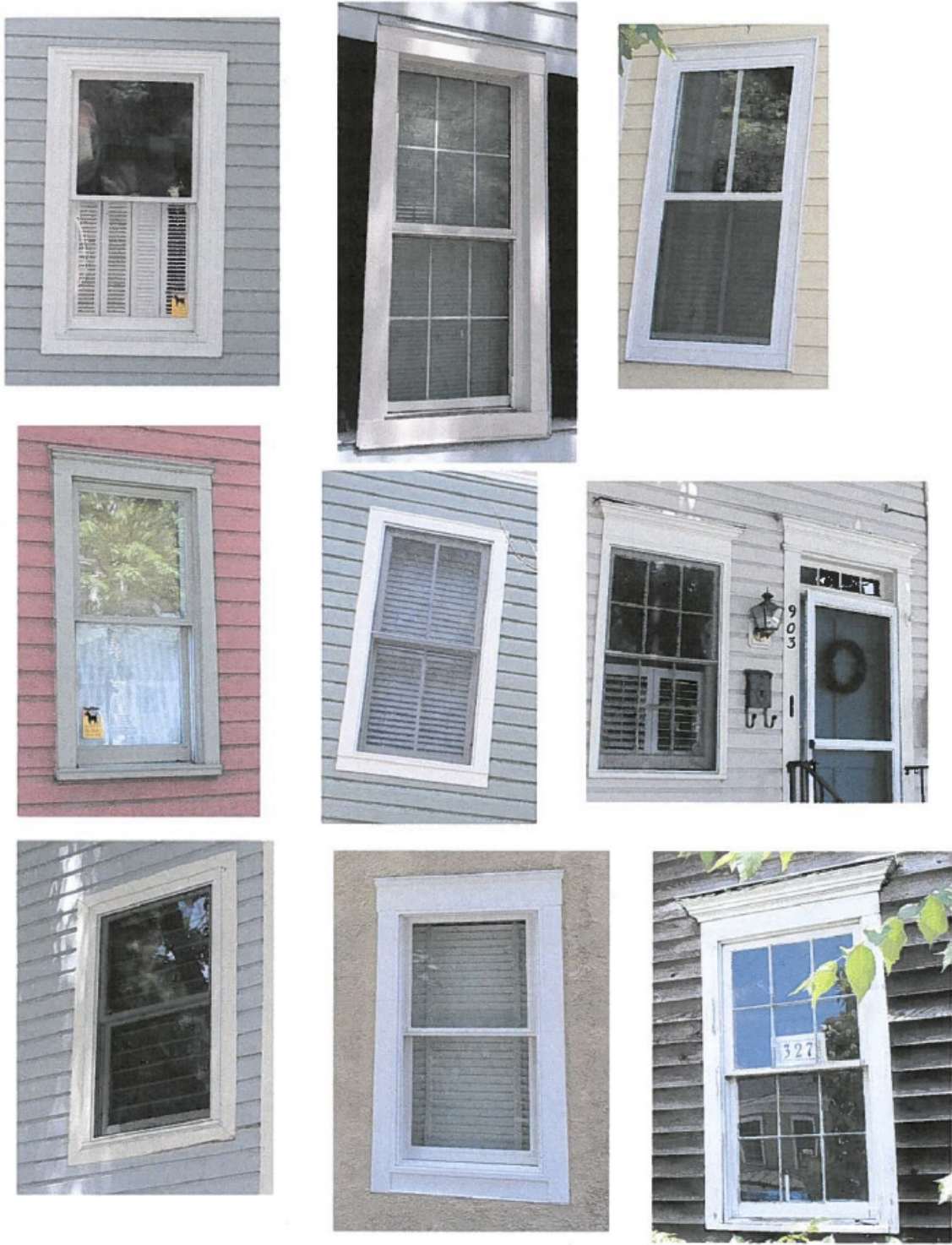
Figure 12. Photos of window trim in the Parker-Gray neighborhood.
