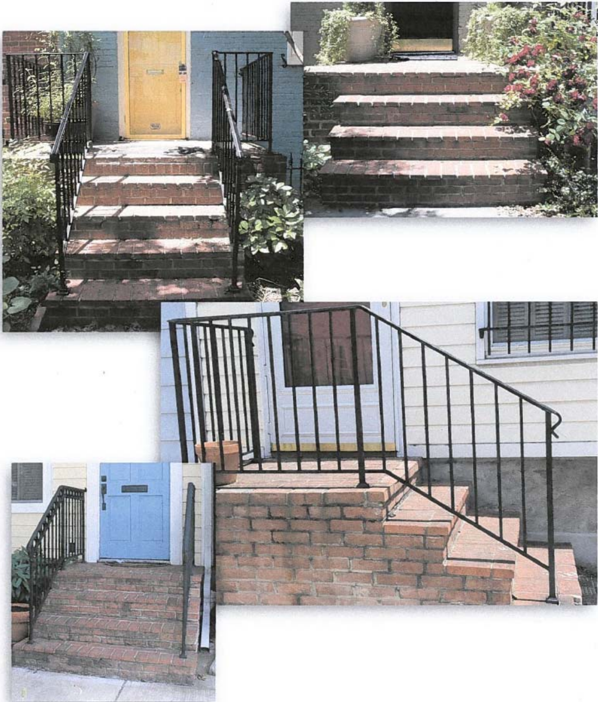
Figure 7. Photos of stoops and railings in the Parker-Gray neighborhood.
