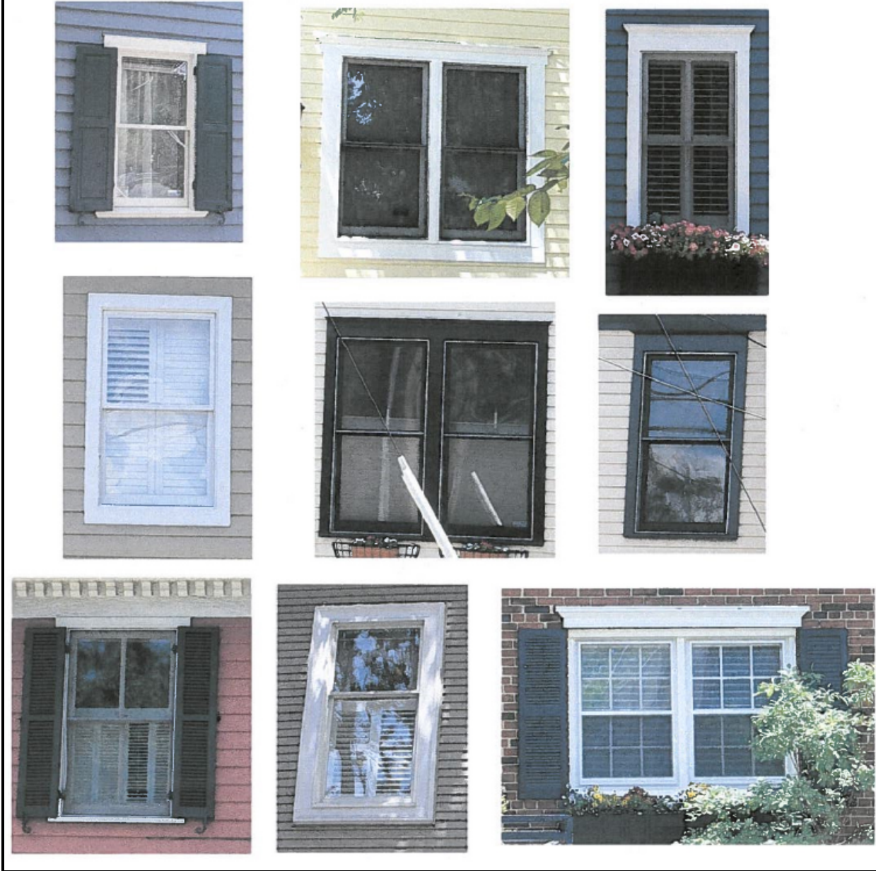
Figure 11. Photos of window trim in the Parker-Gray neighborhood.
