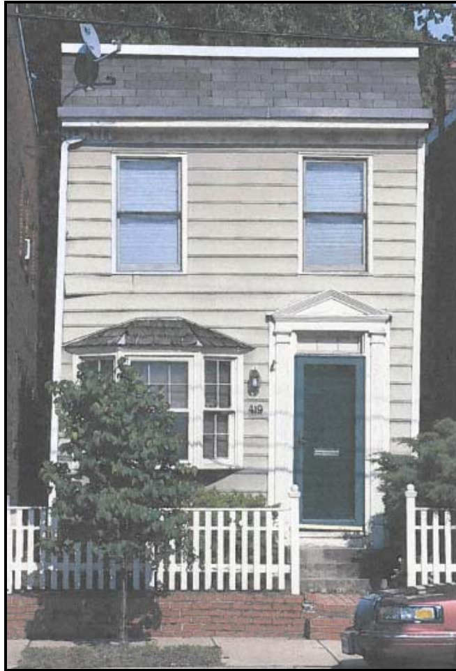
Figure 1. Existing front façade.
