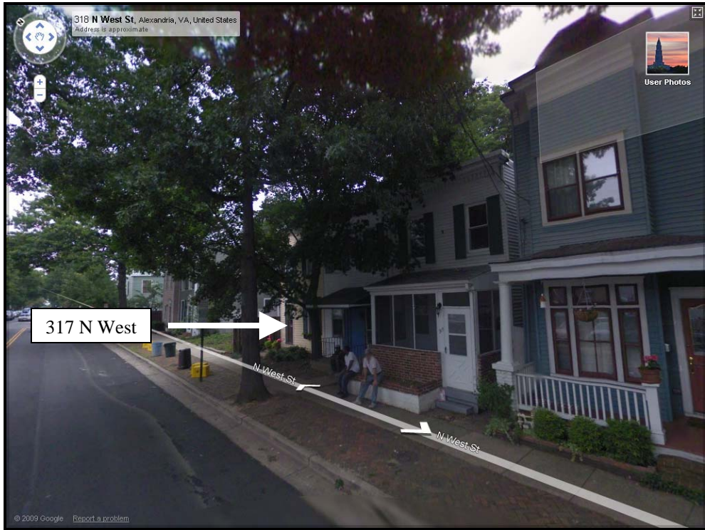
Figure 1. Photograph depicting the porch at 317 N West St prior to removal.
