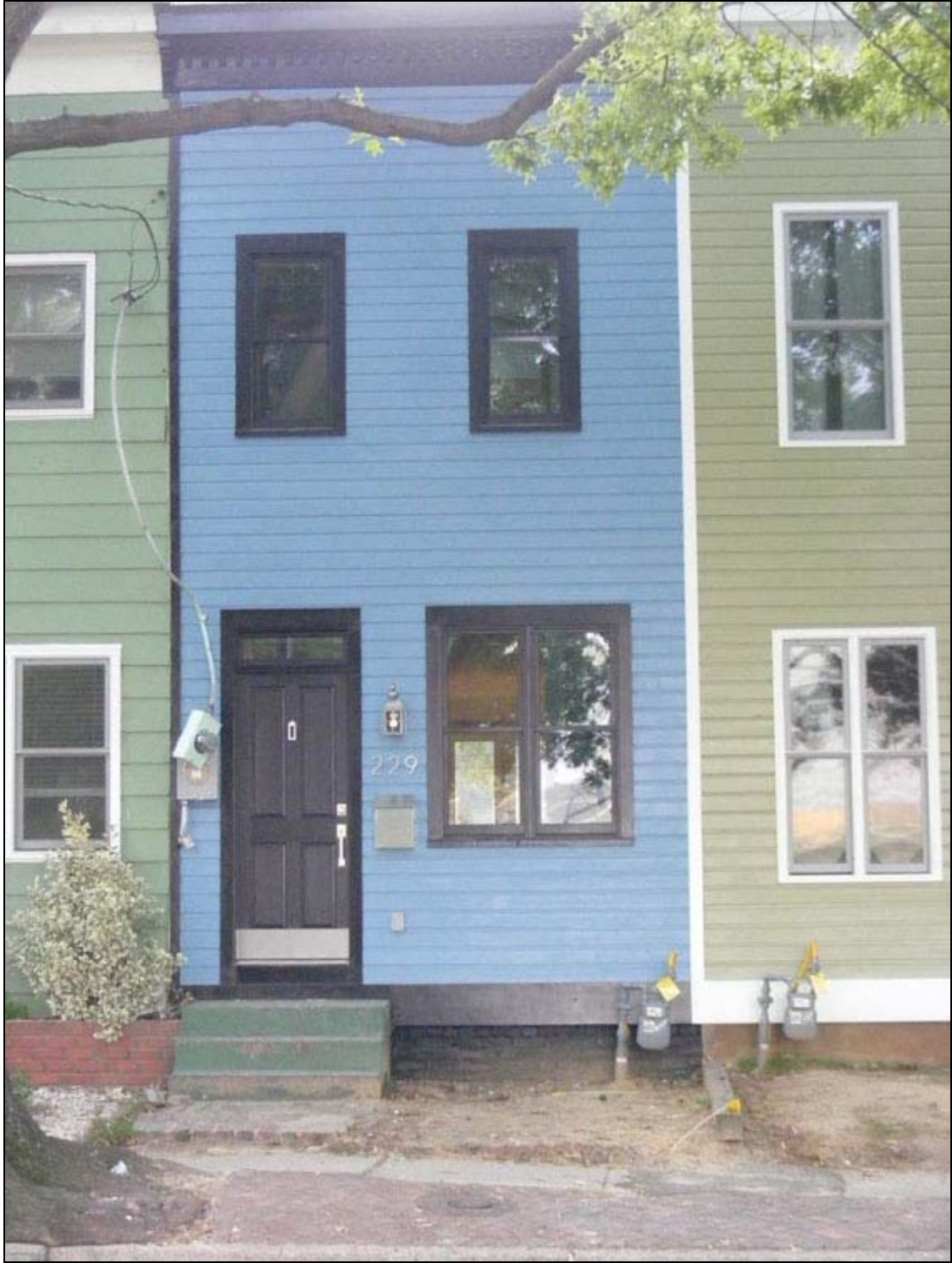
Figure 2. Current front (west) elevation.
