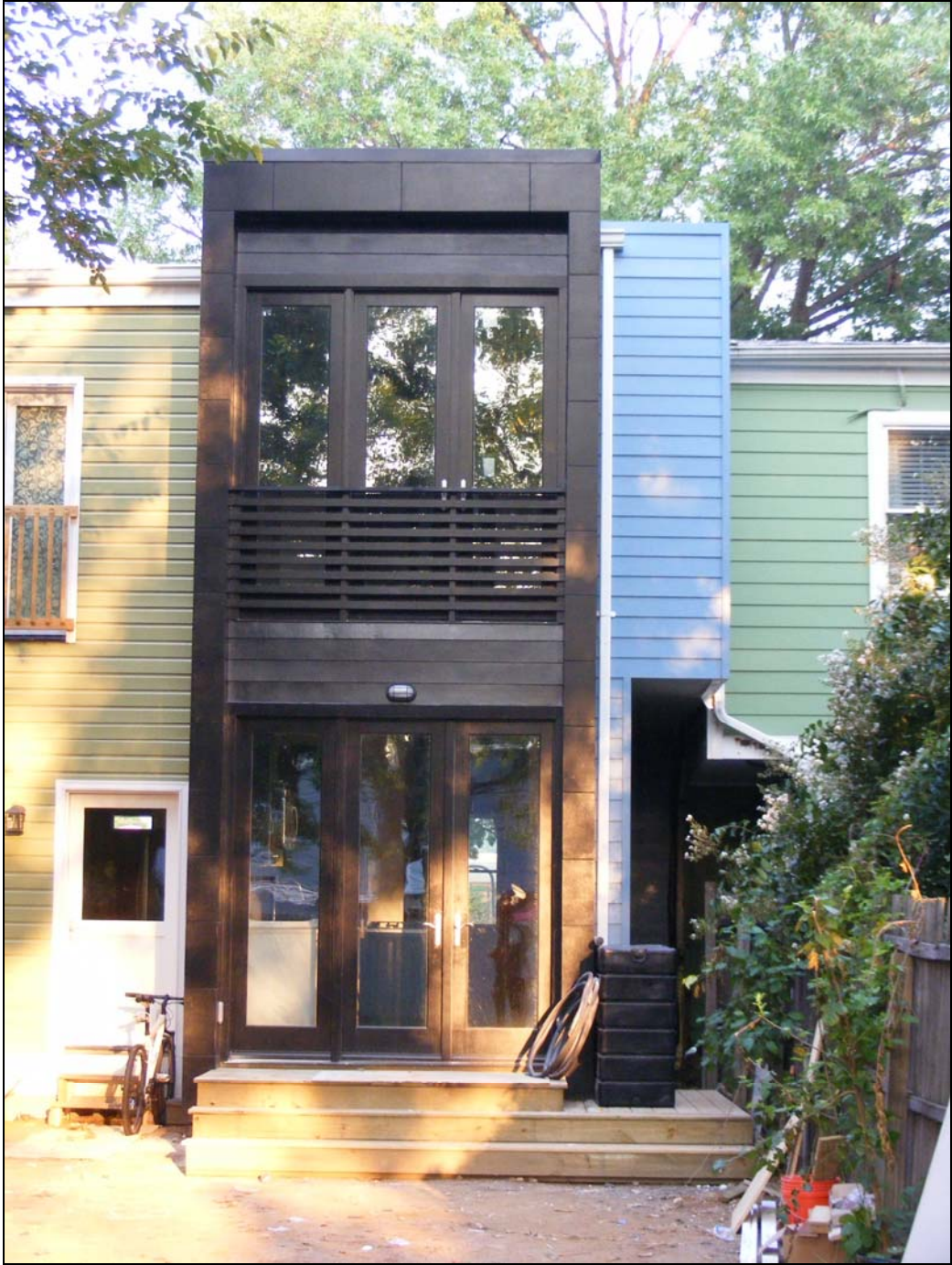
Figure 3. Current rear (east) elevation.
