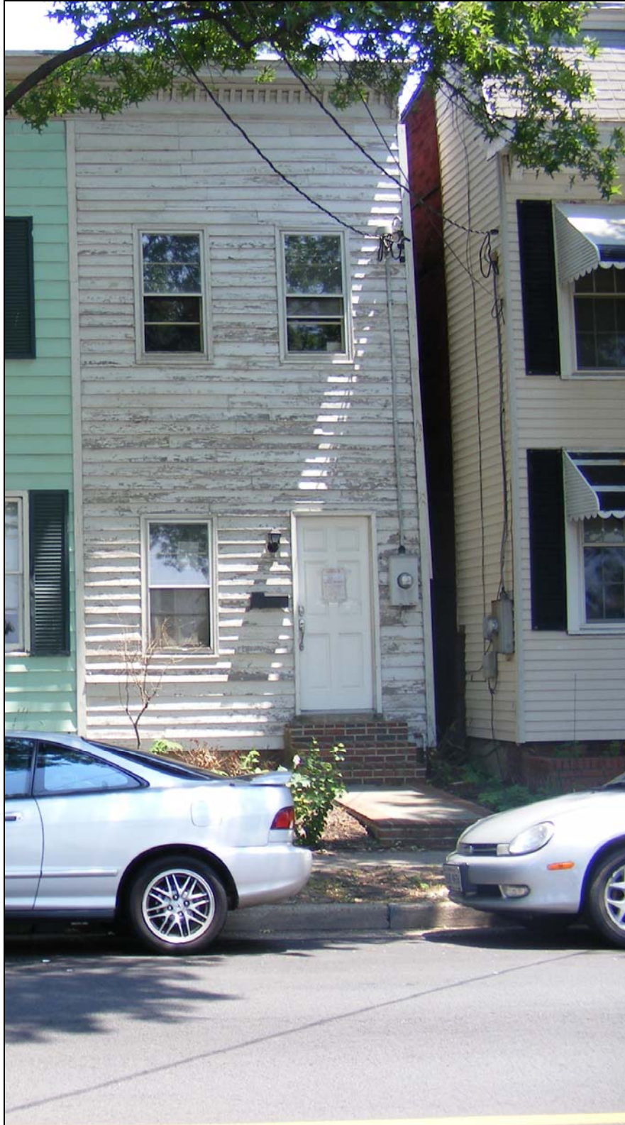
Figure 3. Front (west) elevation showing historic wood siding in good condition.
