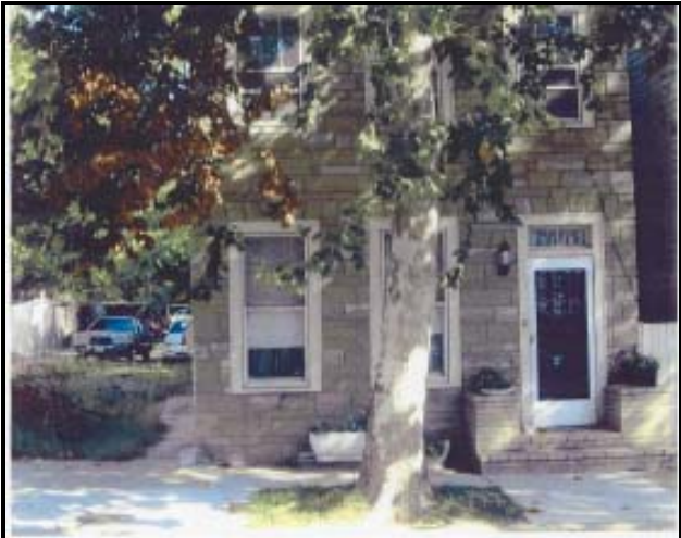
Figure 1: Photo of front elevation.
