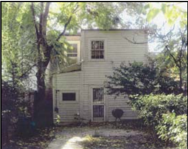
Figure 3: Photo of rear.
