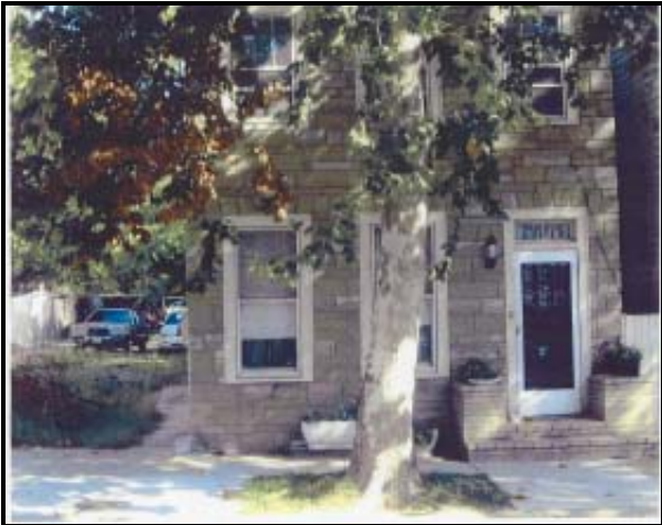
Figure 1: Photo of front elevation.
