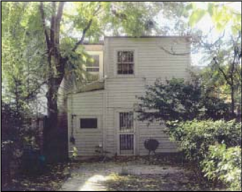
Figure 5: Photo of rear.
