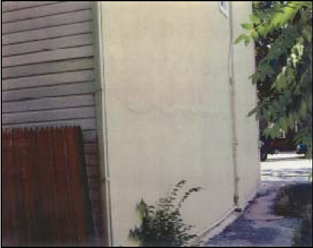
Figure 4: Photo showing side and rear elevations.
