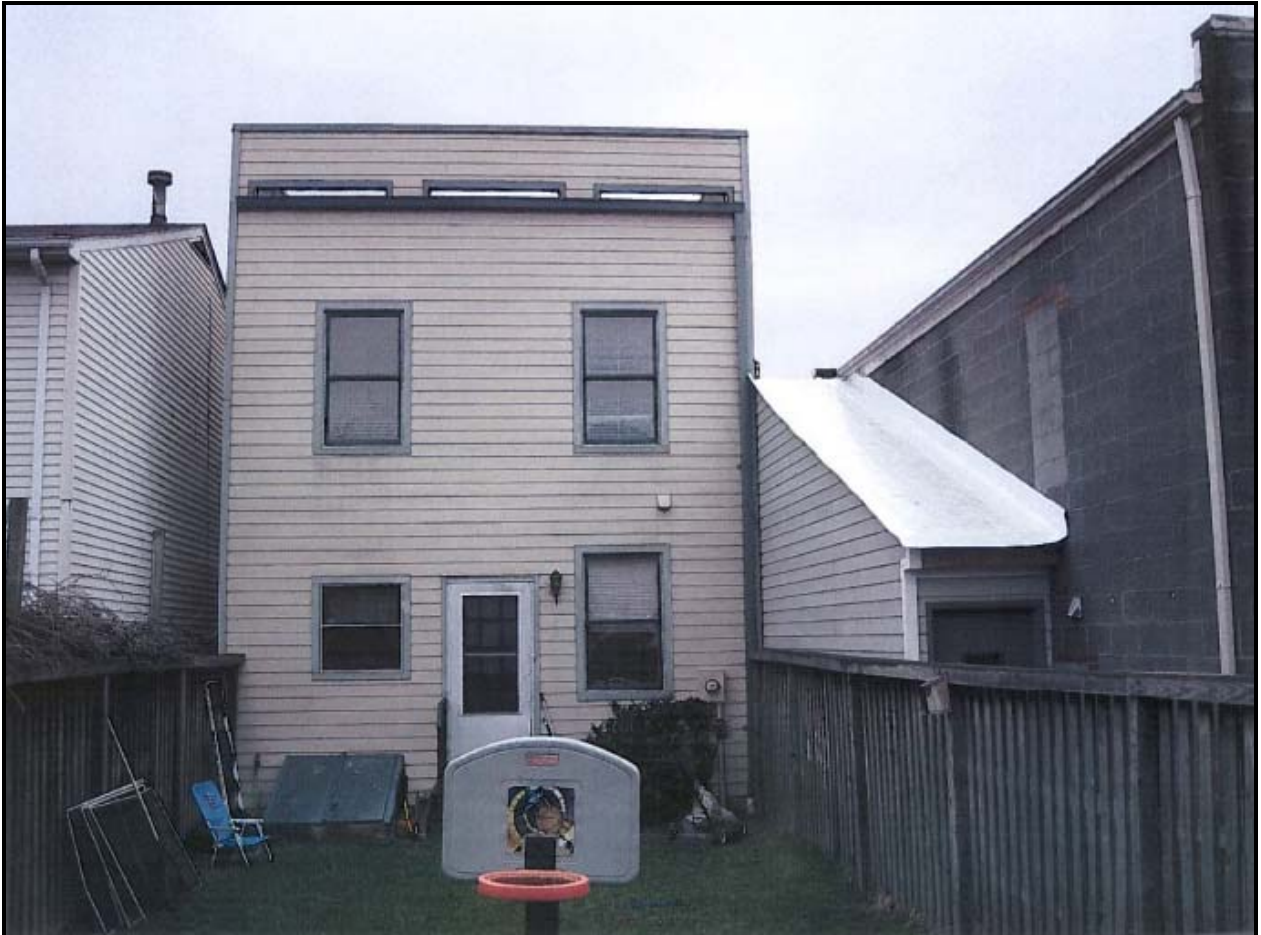
Figure 4: Rear Elevation View of 702 North Patrick Street from inside fenced yard
