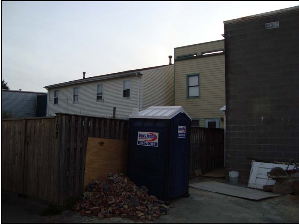
Figure 6: Photo showing rear elevations of buildings that flank 702 North Patrick Street
