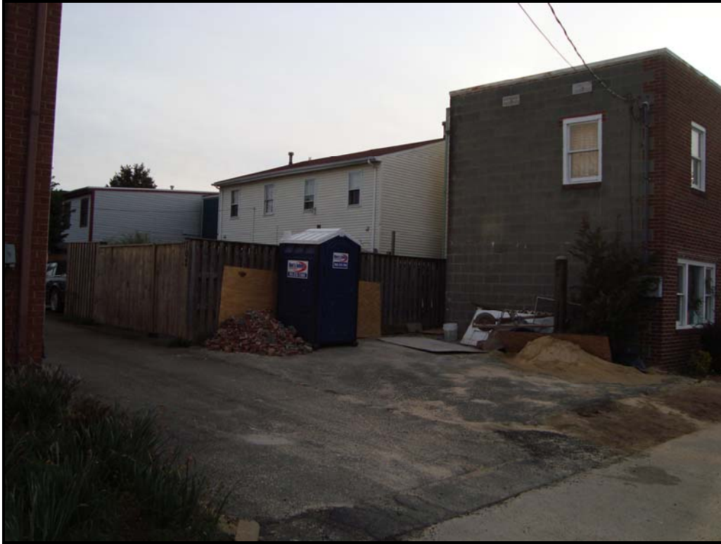
Figure 5: Photo taken from emergency alley entrance on Wythe Street
