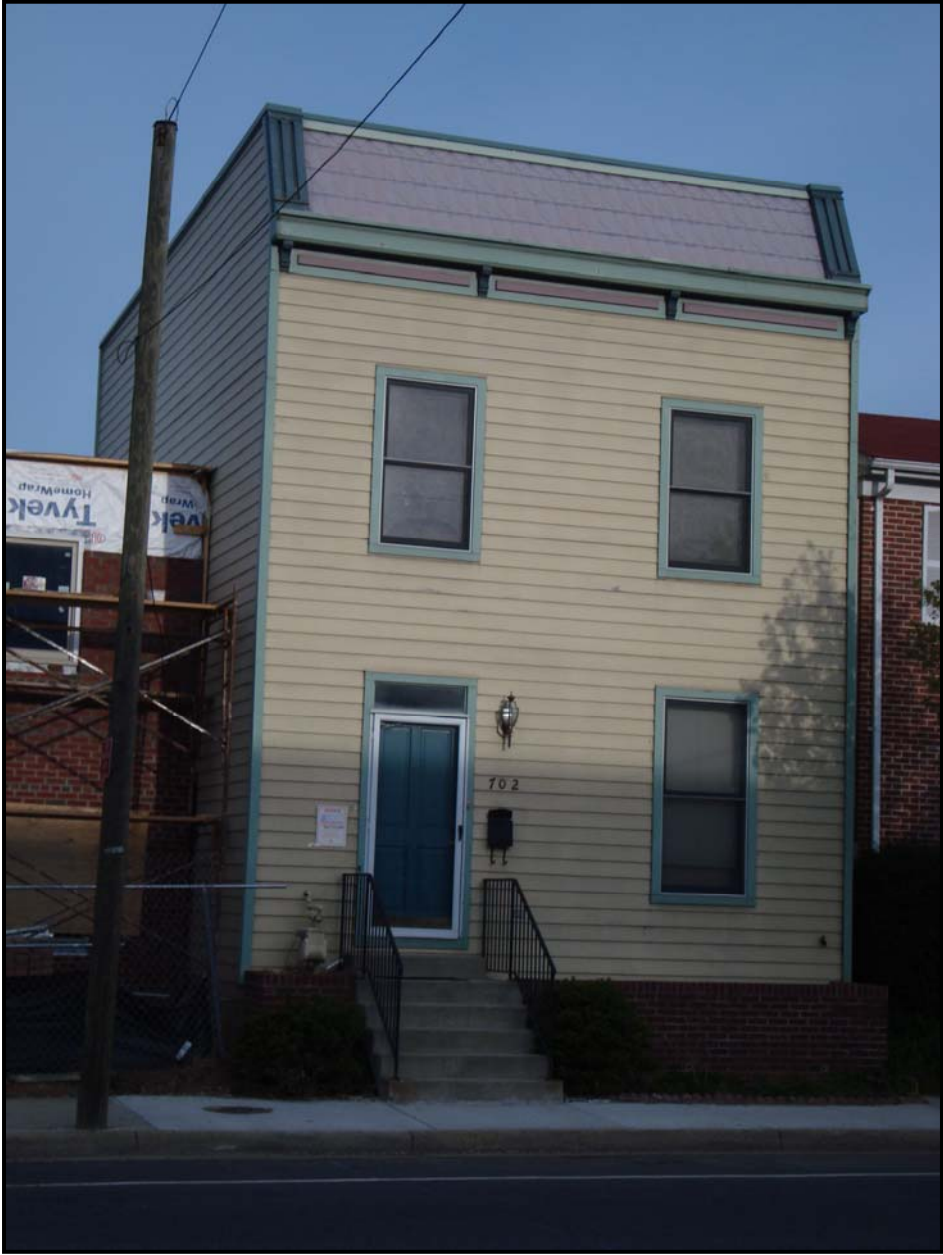
Figure 2: Photo showing of Front Elevation of 702 North Patrick Street
