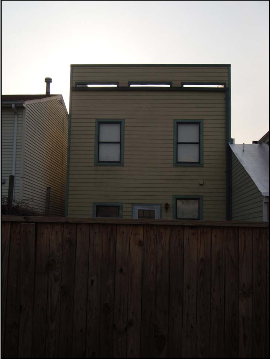
Figure 3: Photo showing Rear Elevation of 702 North Patrick from Alley
