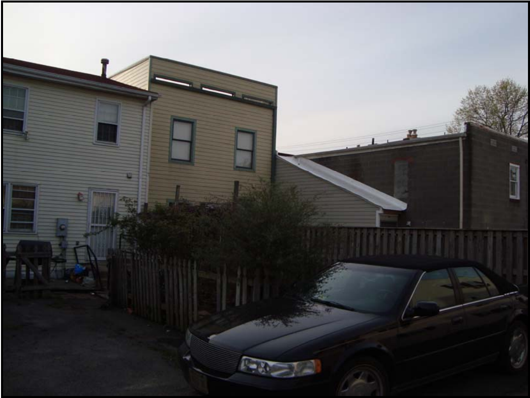
Figure 7: Photo showing rear elevations of buildings that flank 702 North Patrick Street
