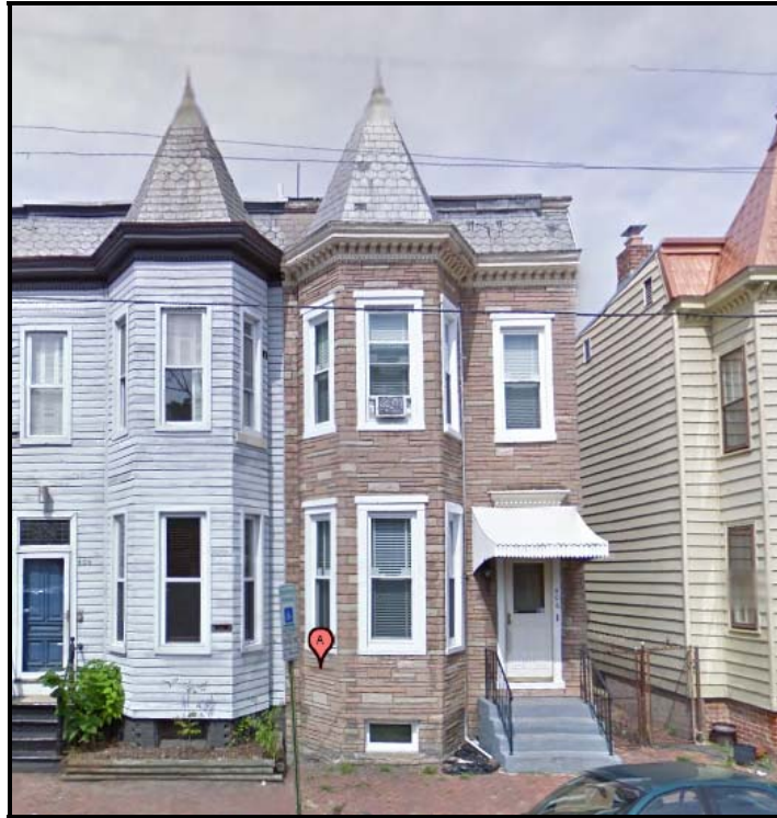
Figure 1. Photo of Existing Conditions – Front Elevation
