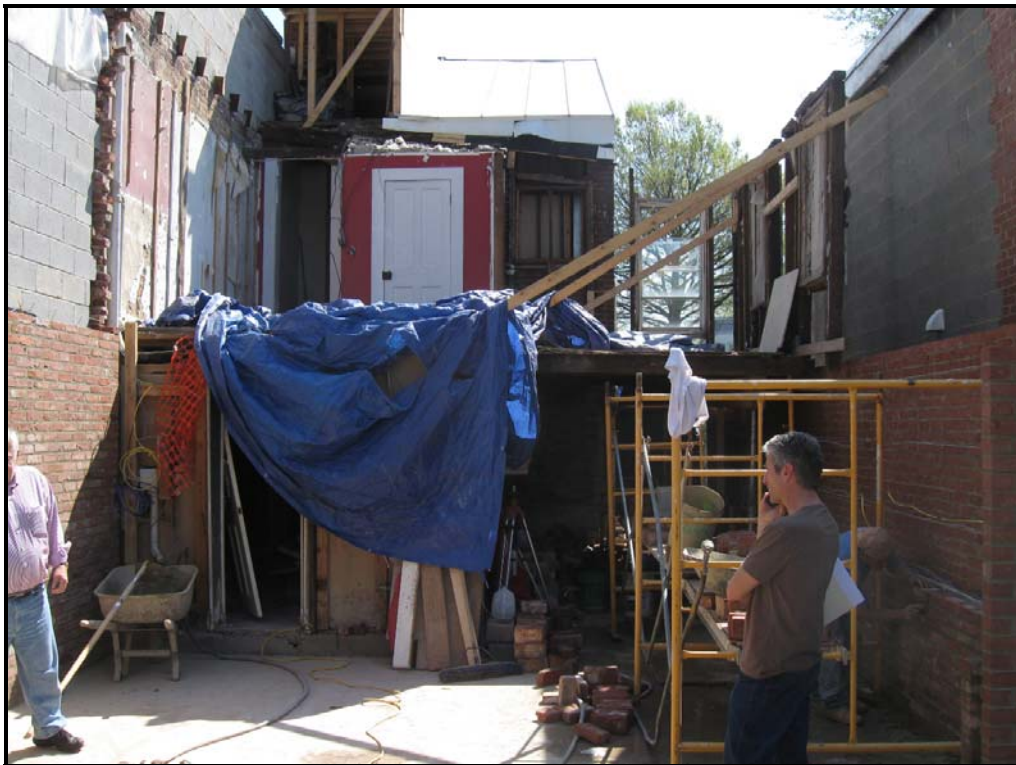
Figure 2. Existing Condition Photos
