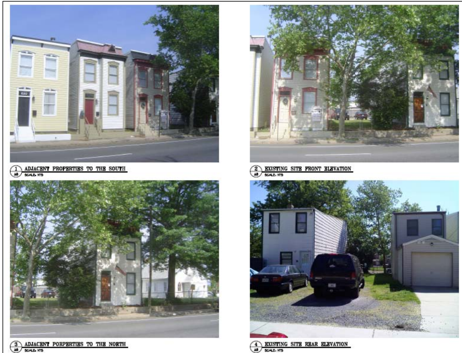
Figure 1. Existing buildings and conditions.
