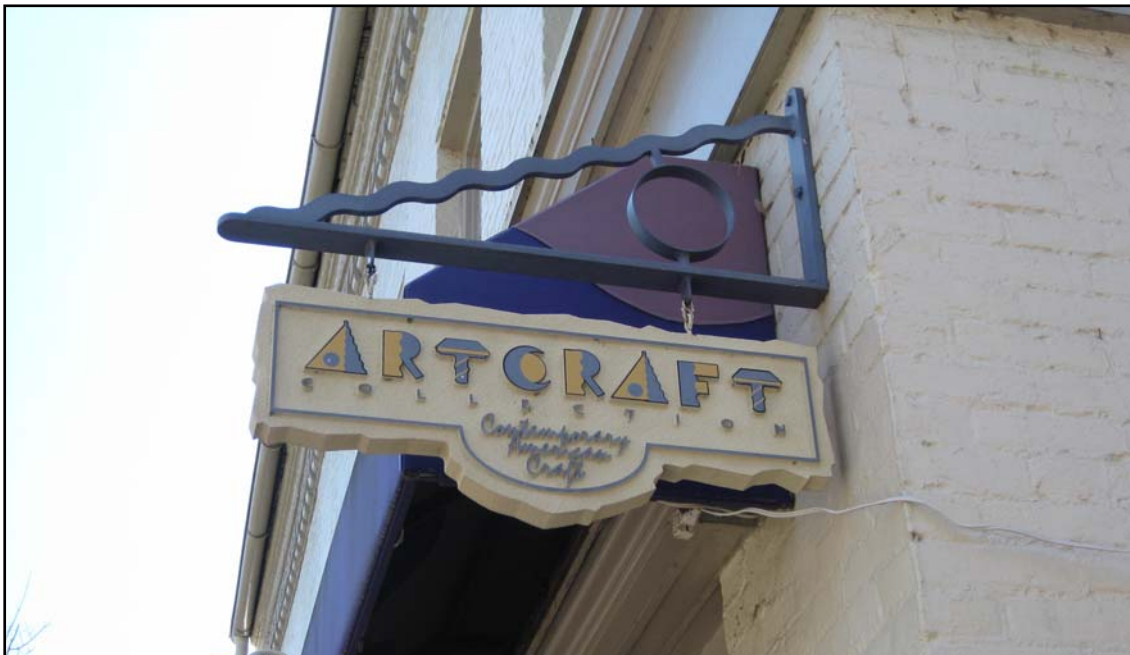
Figure 6: Existing HDU sign installed 10 years ago in excellent condition.
