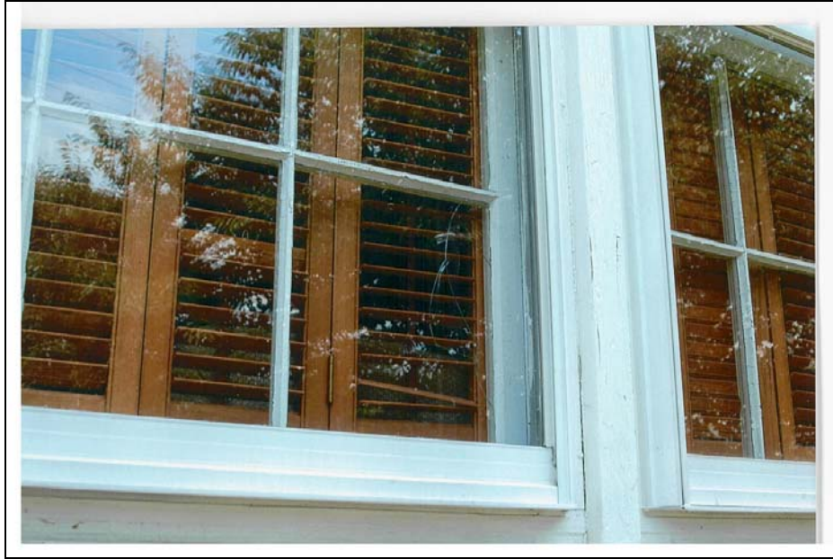
Figure 3. Detail of existing window.
