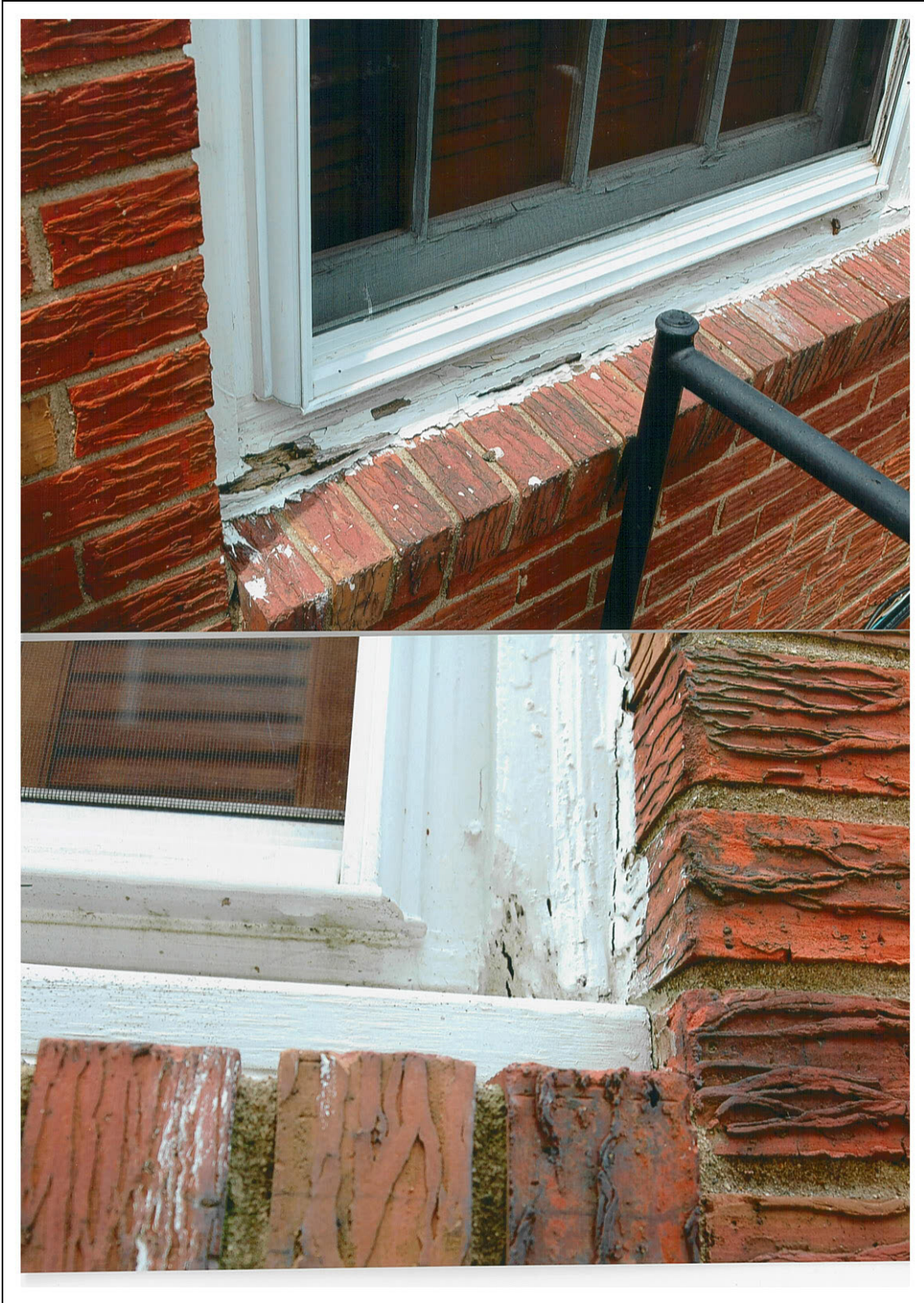
Figure 2. Details of existing windows.
