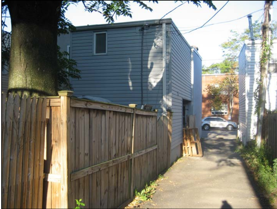
Figure 3. Rear (east) and side (north) elevations.
