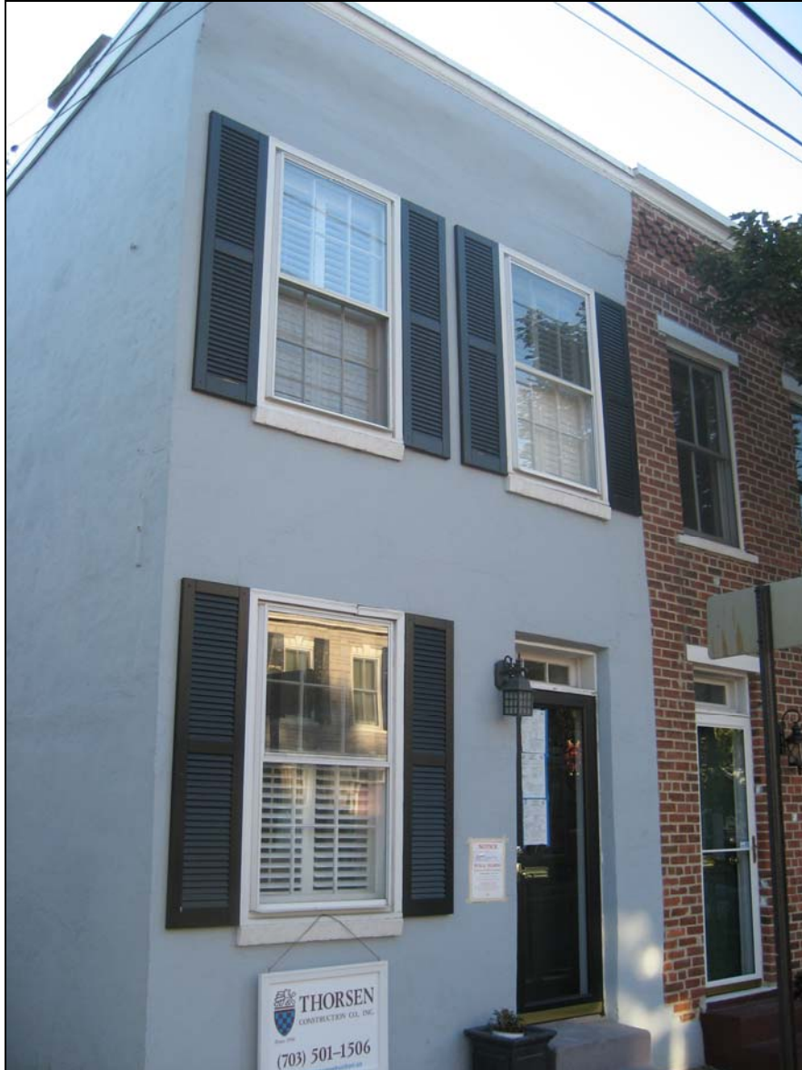
Figure 2. Front (west) elevation.
