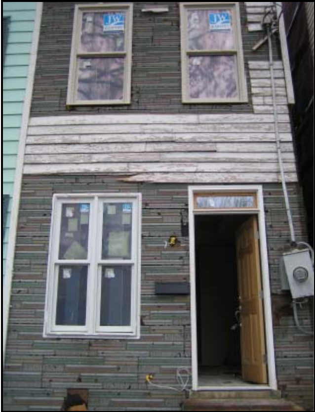
Figure 12: Applicant’s photo showing wood siding over Insulbrick.
