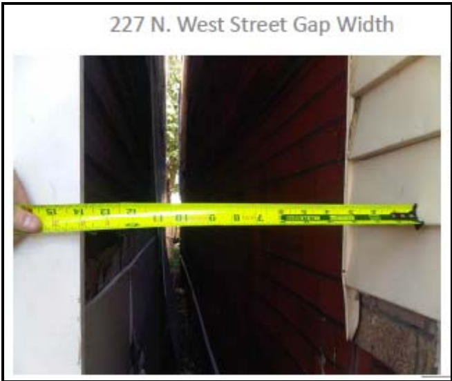
Figure 5: Photo showing 14” width of opening between houses.
