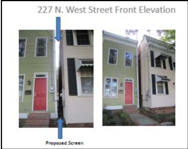
Figure 4: Photo of front façade showing gap between houses.
