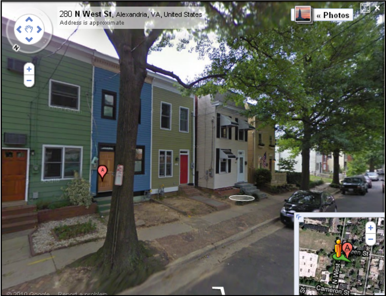
Figure 1. Google maps image of 227 North West Street and neighboring properties.
