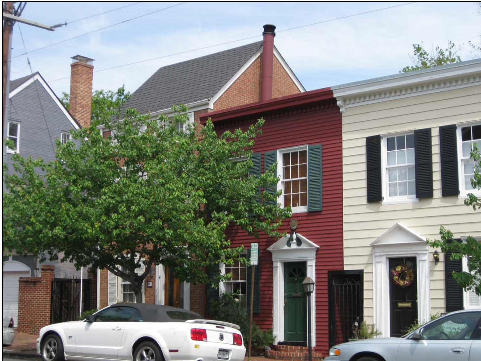
Figure 5. Example of a similar flue extension in the Old and Historic Alexandria District.
