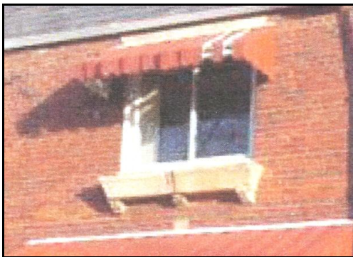
Figure 2: View of planter box before removal.
