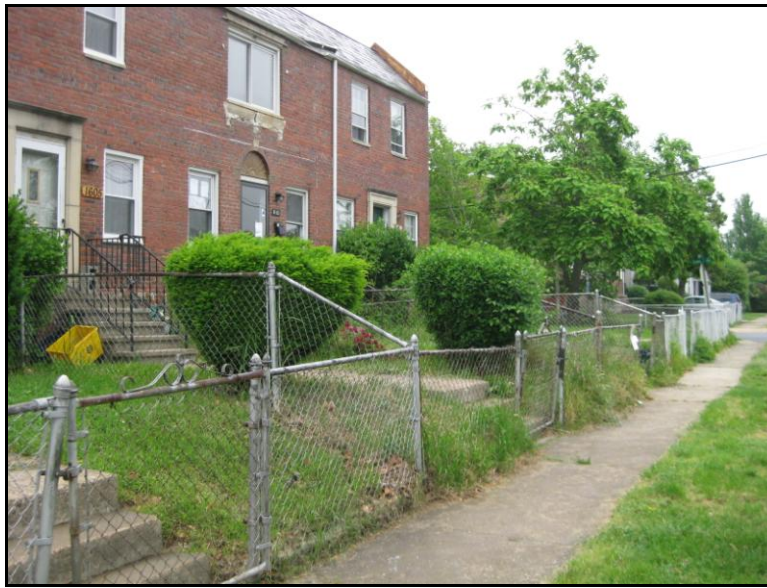
Figure 4: View of cohesive streetscape of chain-link fencing along Princess Street.
