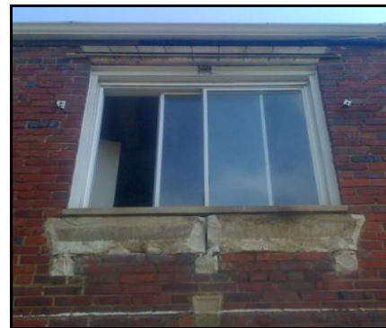
Figure 3: View of planter box after removal.
