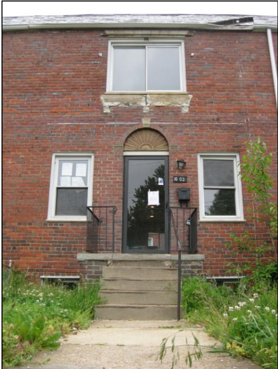
Figure 6: Current view of 1603 Princess Street after removal of planter box and metal awnings.
