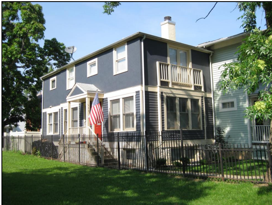
Figure 3: West and South elevation of 1403 Princess Street. Note: the metal fence in the foreground is a neighbor's property line fence.
