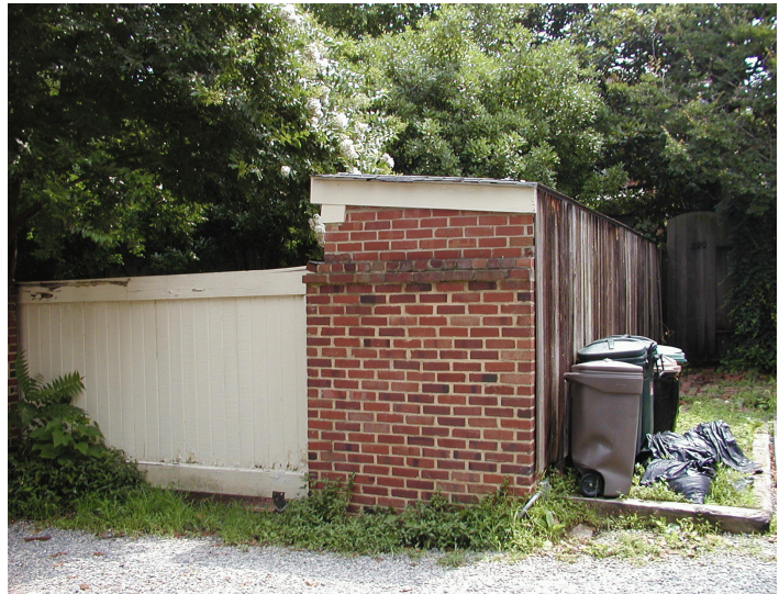
Existing one-story brick storage shed
