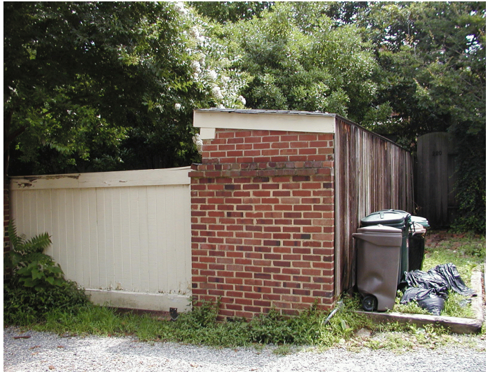
Existing one-story brick storage shed
