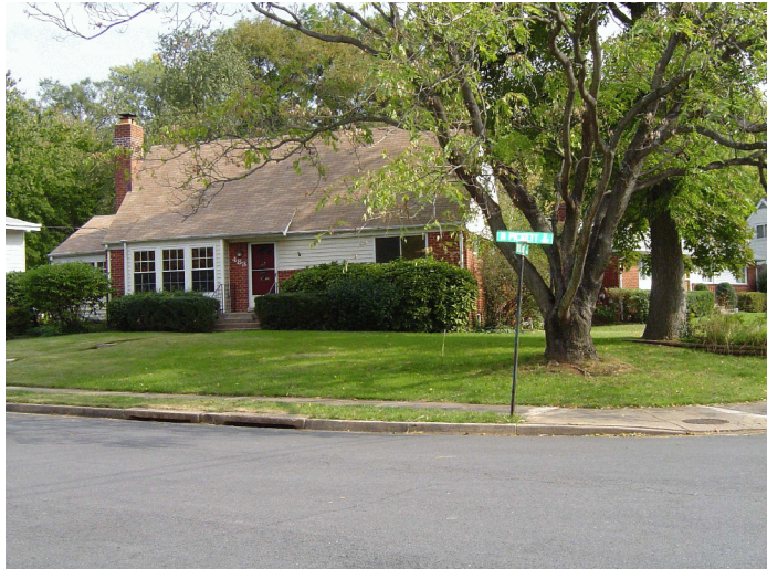
Existing house at 483 North Pickett Street
