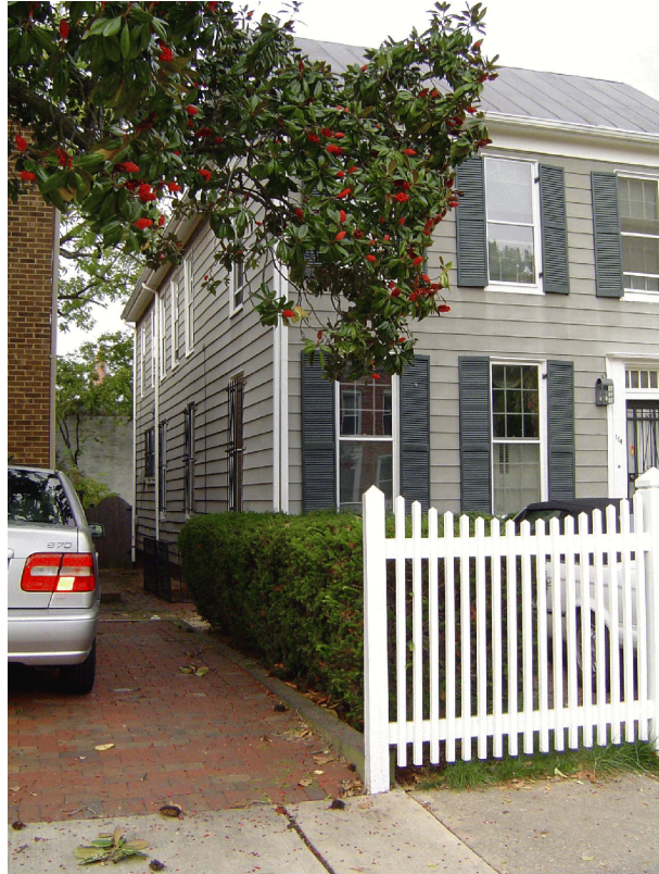
Existing house at 114 North Payne Street
