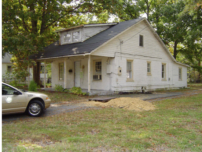
Existing vacant house at 5300 Seminary Road
