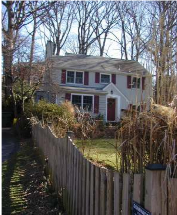
Figure 1- View of north side yard from Russell Road
